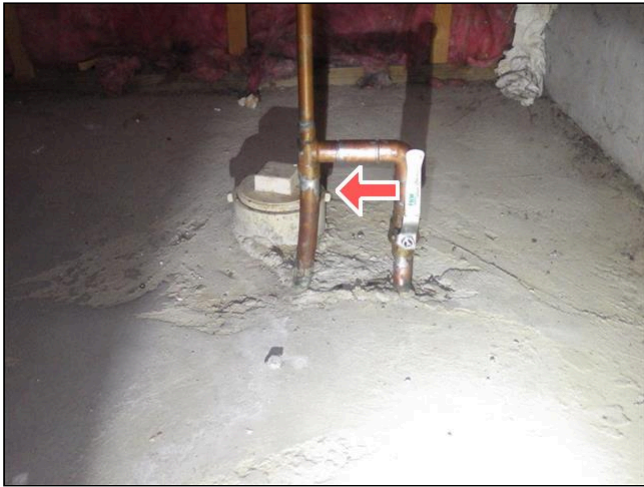
Basement - Under the Stairway
